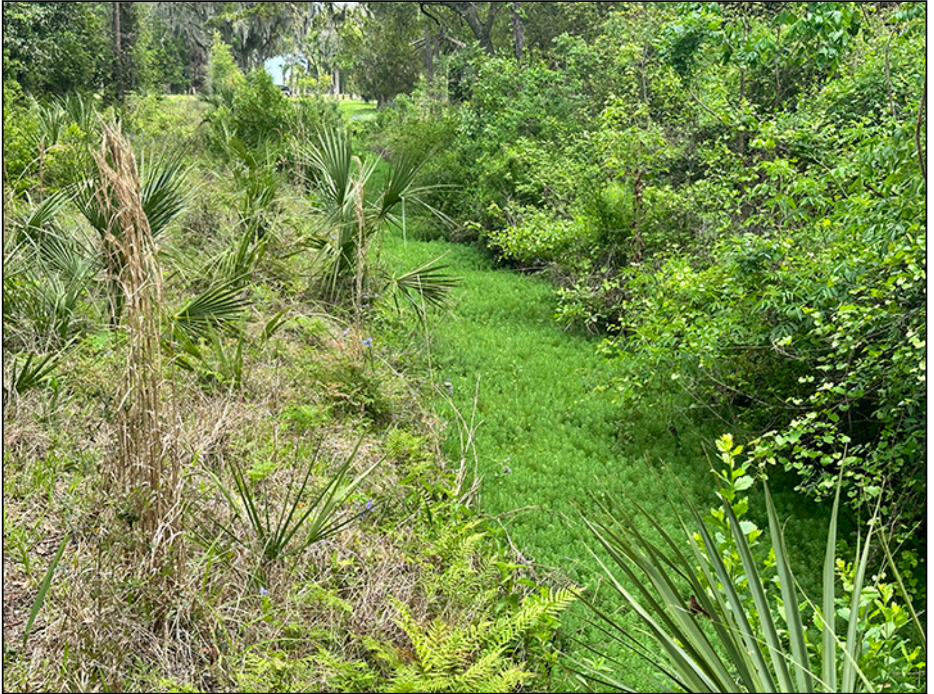
Figure No. 8 - Overall condition of the Drainage ditch needing maintenance with woody stem vegetation leaning over the system from the South bank.
